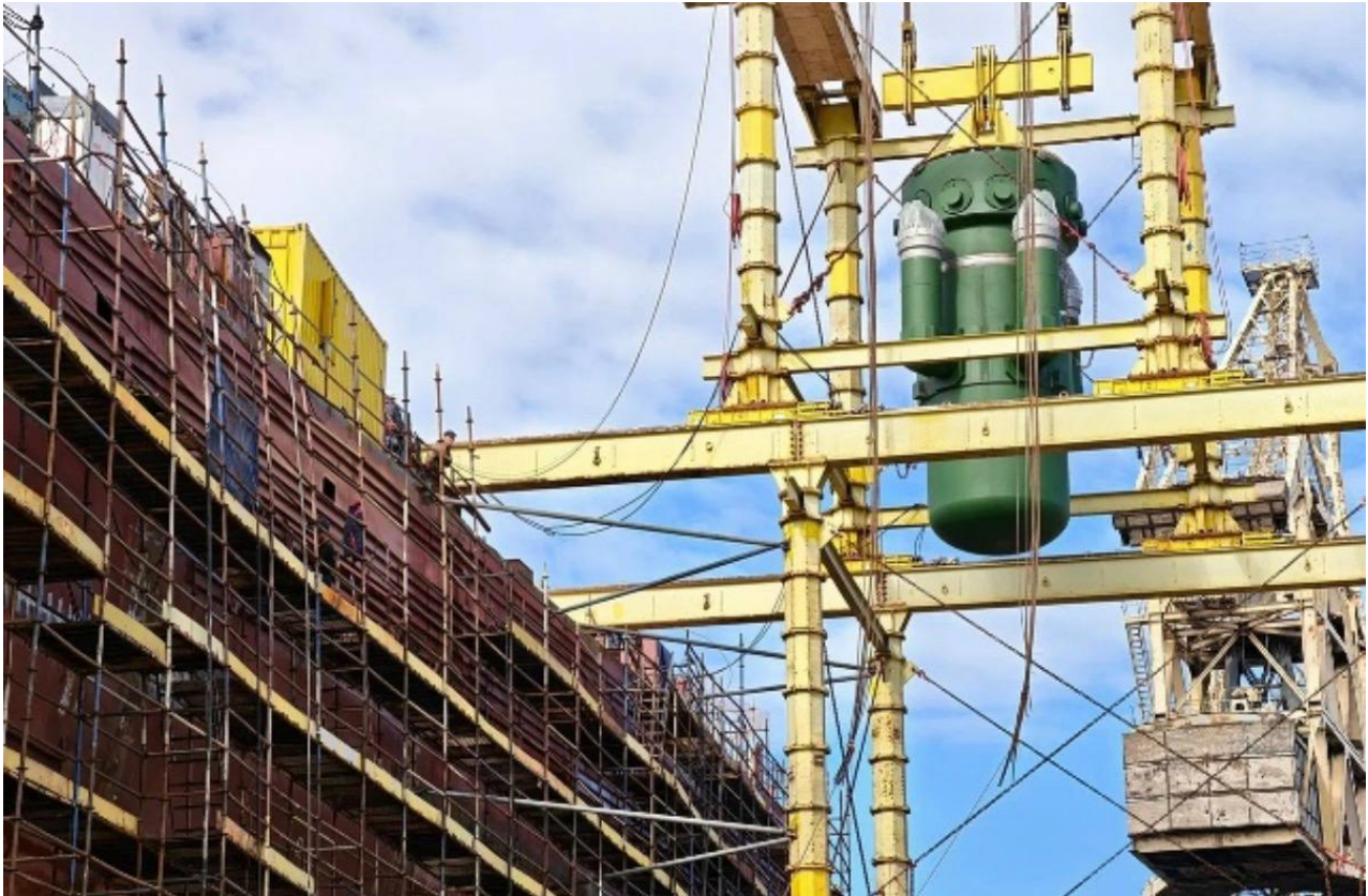
Nuclear reactor installation on the Leningrad icebreaker under construction.
