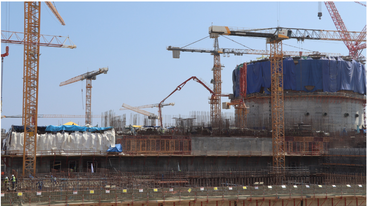
Unit 1 of the El Dabaa NPP under construction, Egypt.
