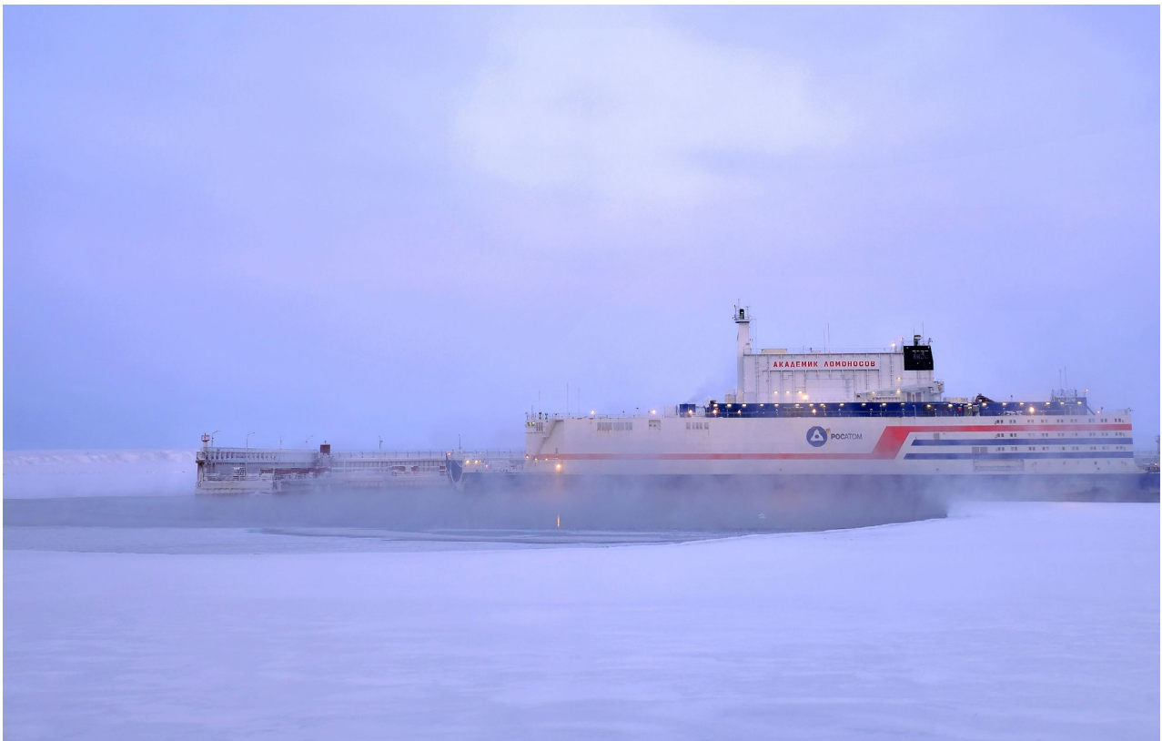
Akademik Lomonosov floating nuclear power plant.
