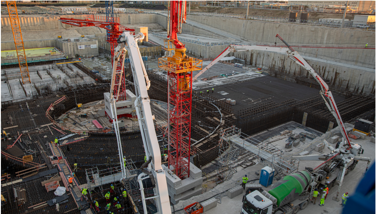
Start of construction of the reactor building foundation slab for Unit 5 of the Paks II NPP.
