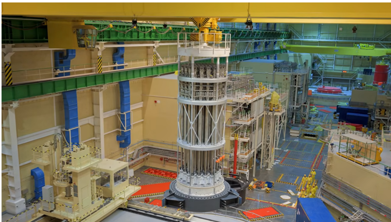
Nuclear fuel loading at Unit 4 of the Mochovce NPP.
