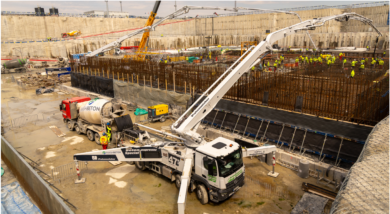
Concreting of the foundation slab for unit 5 of the Paks II NPP.
