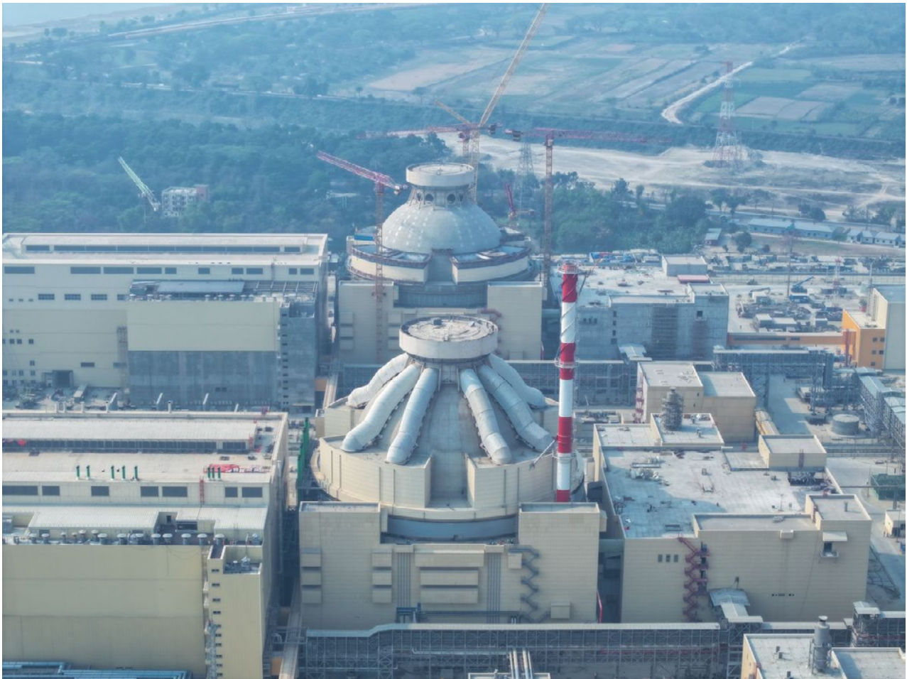
Units under construction at the Rooppur NPP, Bangladesh. Source: Rosatom
