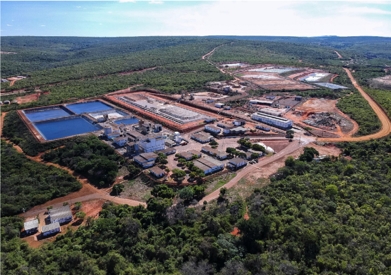
Uranium concentrate production facility in Caetité, Brazil. Source: INB
