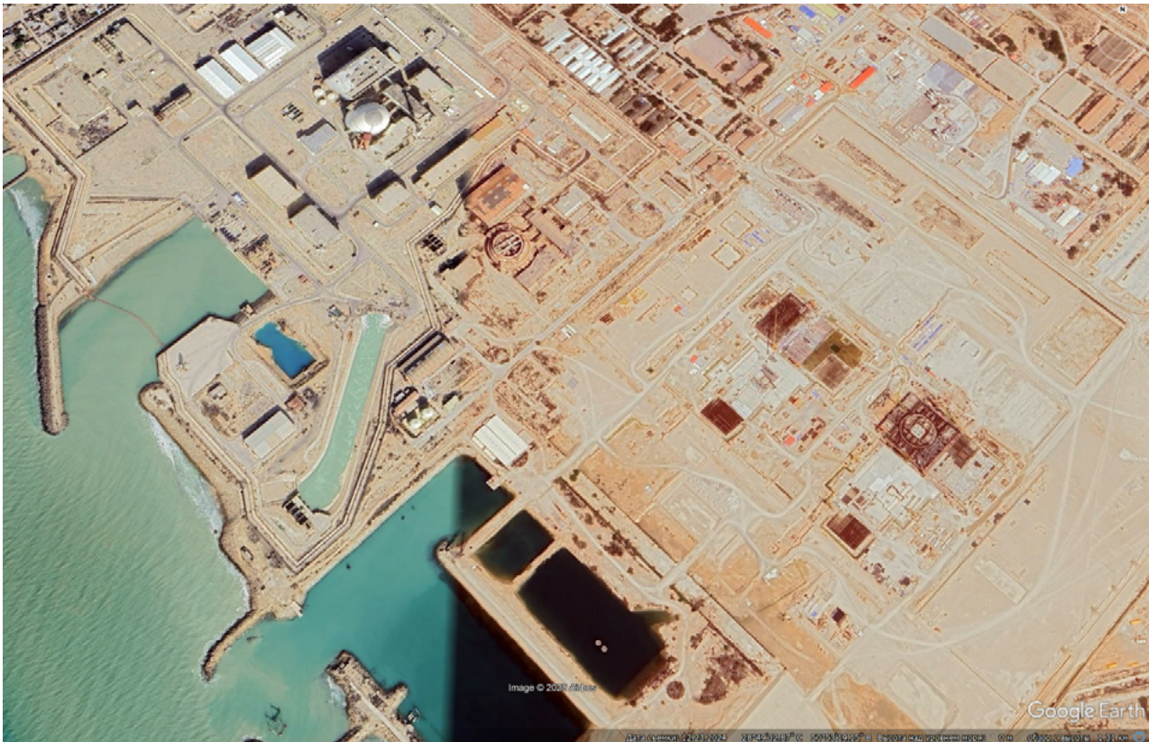
Bushehr NPP. The operating Unit 1 with its white dome is visible in the upper left; the construction site for two new units is in the lower right. Satellite image from Google Maps, 2024. Impact of US-Israeli strikes on Iran
