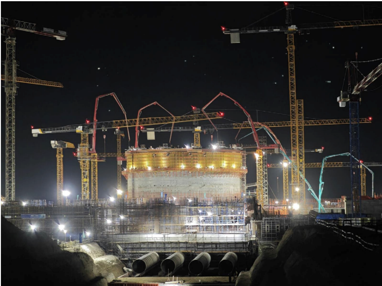
Unit 2 of the El Dabaa NPP under construction, Egypt. Source: ASE 225
