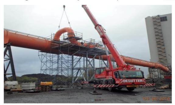
Picture: the gas off take for the steel mill gases, to the fermentation plant have already been installed.
