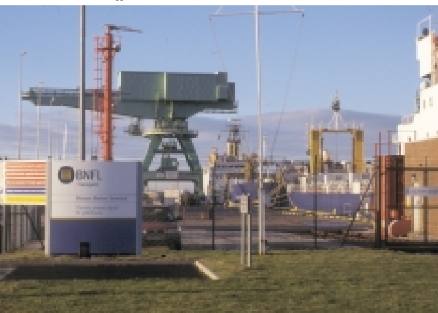
BNFLs kaianlegg i Barrow
