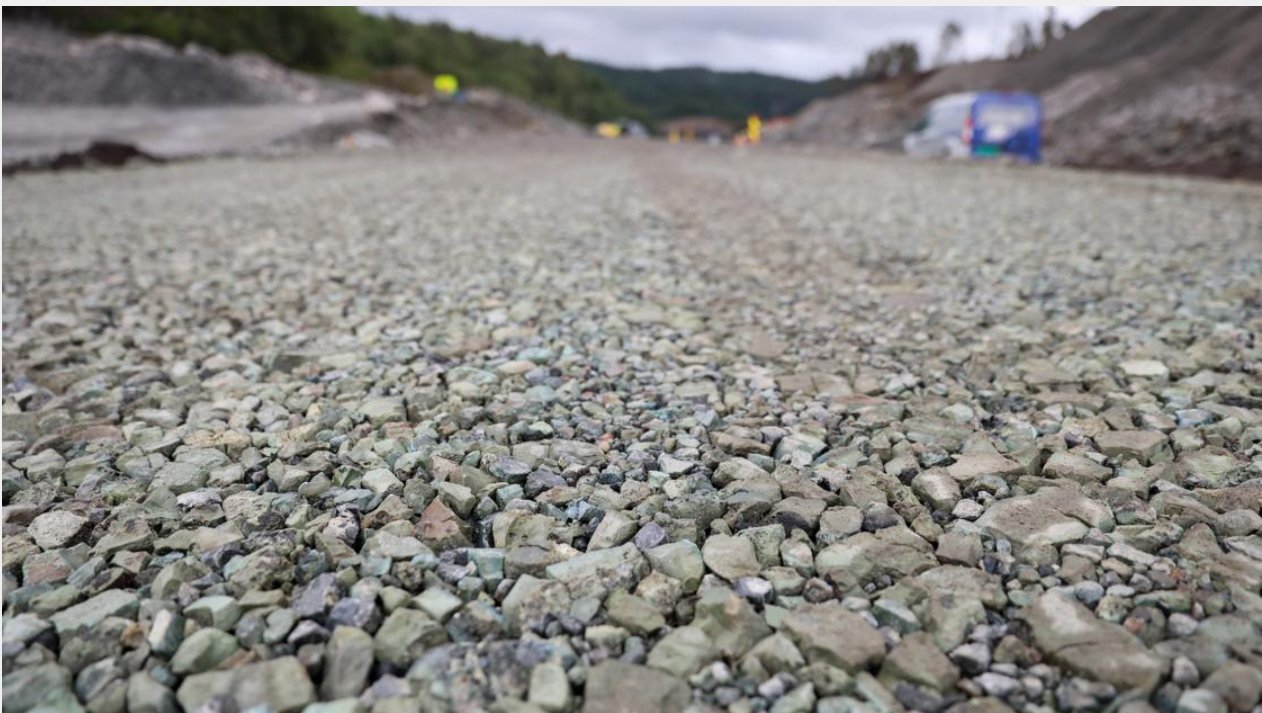
Figure 3: Low carbon material Silica Green Stone, made from waste from Eramet smelter plants, used in construction of the new E39 in Lyngdal. Photo credit: Nye Veier.
