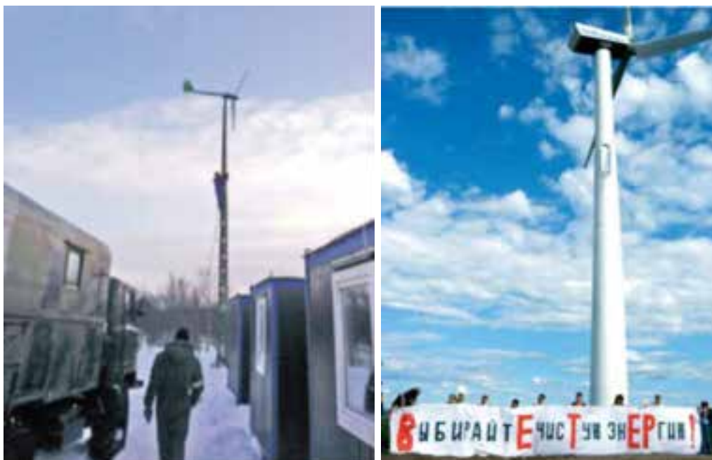
Left: Wind power installation in Novaya Titovka, 9 kW (Foto: ООО «Murmansk»)
